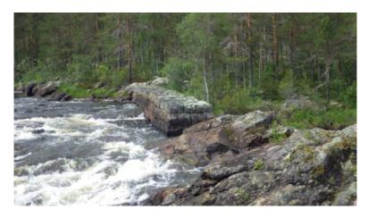
**Figure 10.3:** Historical remains of the log-driving epoch include built-up banks along the river. The picture shows a particularly substantial stone banking at the Hylströmmen rapids. Photography: Anders Persson/Linda Jonsson
