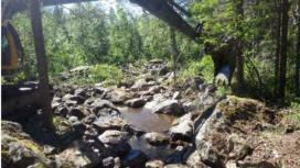
**Figure 3.8:** Restoration of Kalvsån river, previously cleared for log driving. To the left, the river straightened for the transportation of timber; to the right, the same river during the restoration process. Photography: Peter Hallgren, Fiskevårdstjänst.
